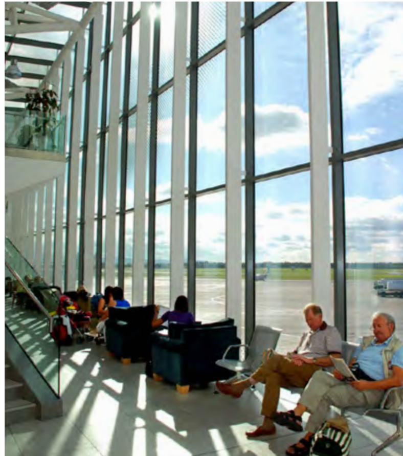
Pictured above: The Terminal 1 Arrivals Refurbishment Project was designed such that the existing façade was modified to optimise the use of natural light to reduce internal lighting requirements.
